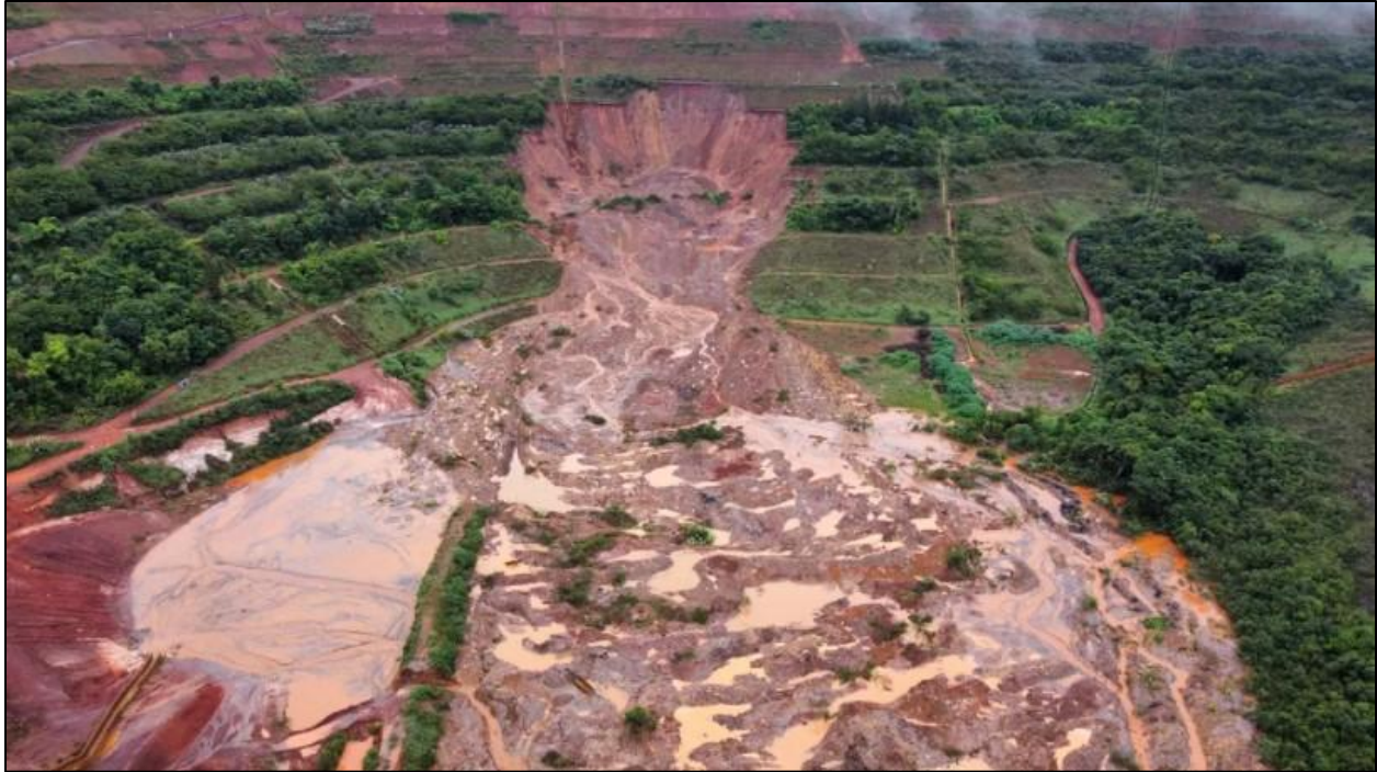
Figure 7. A 48-meter-high filtered tailings stack at the Pau Branco iron-ore mine in Brazil collapsed on January 8, 2022, due to heavy rain. Although filtered tailings are regarded as the Best Available Technology at the present time (Morrill et al., 2022), the failure of a filtered tailings stack should not be regarded as impossible, especially in areas with high precipitation. Photo from Angelo (2022).
